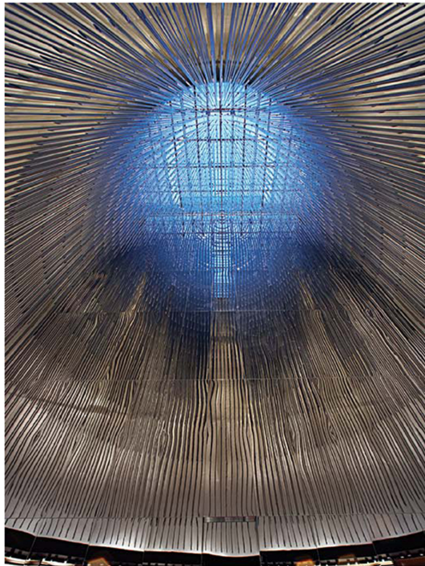
The central atrium in the Louis Vuitton Champs Elysees building in Paris is composed of 2000 stainless steel rods suspended above the skylight in a half-dome pattern.
